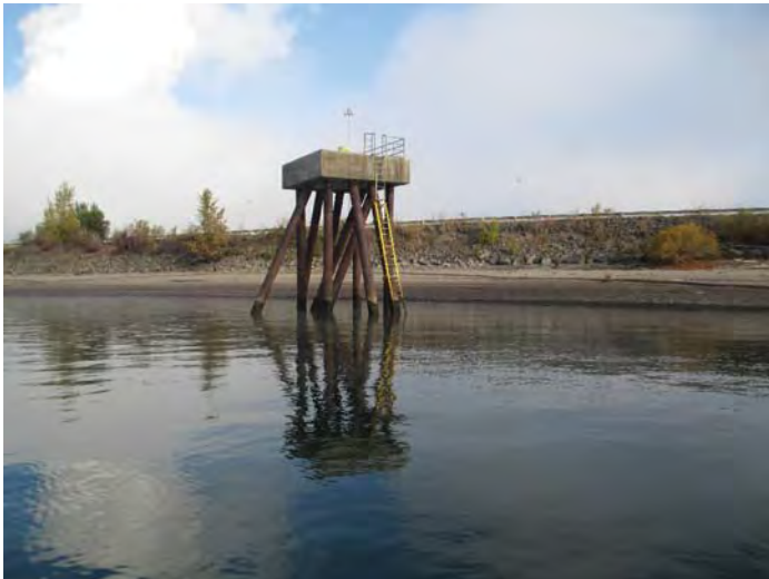
Photo 3: Existing Mooring Dolphin
