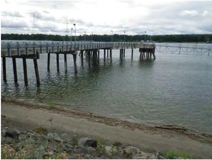
Photo 1: Existing Berth 13 Trestle and Dock
