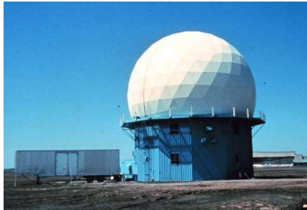
Figure 13. First NEXRAD WSR-88D radar, Norman, OK
