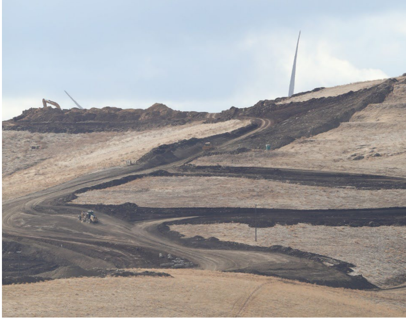
Photo 1. Construction grading for a repowered wind project destroyed every ground squirrel burrow complex encountered, which also diminished breeding opportunities for burrowing owls and forage for golden eagles, September 2019. This view includes only two wind turbine pads; the rest of the grading was for access roads.
