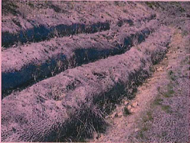
ELK TRACKS ON JUTE ROLLS. NOTE GRASSES GROWING THROUGH JUTE MATS. R LATHAM WHWF 4-16-15
