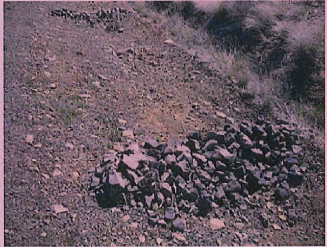
SEDIMENT HAS BEEN CLEANED OUT FROM THIS ROCK CHECK DAM. R LATHAM WHWF 4-16-15
