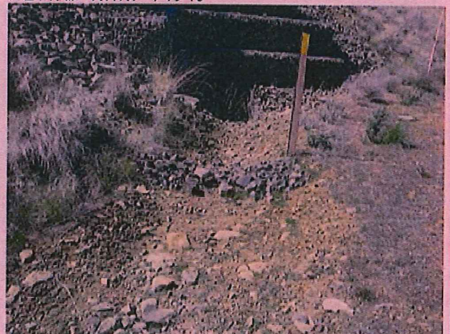
THIS CHECK DAM COULD USE A CLEANOUT. R LATHAM WHWF 4-16-15
