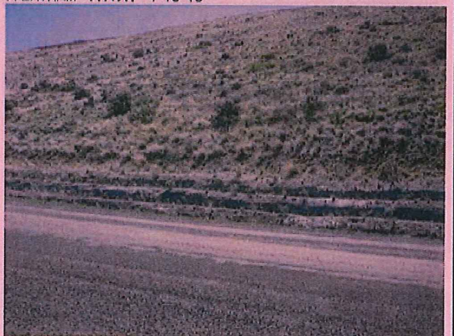
THE JUTE ROLLS STABILIZE THE TOE OF THE SLOPES. R LATHAM WHWF 4-16-15
