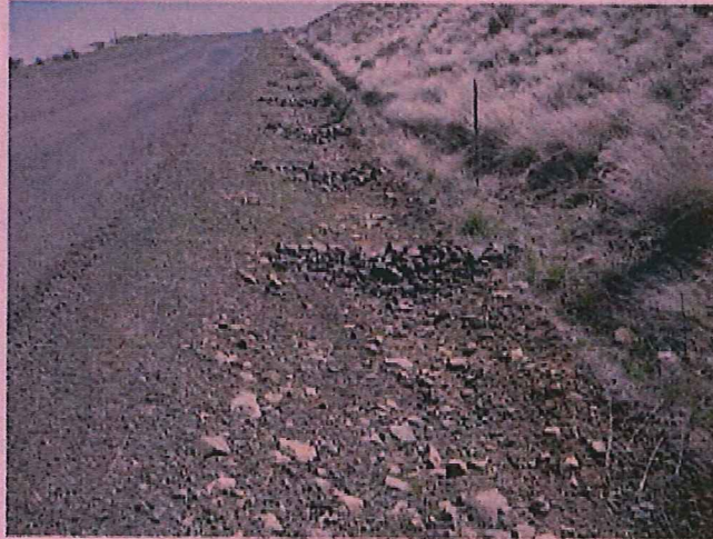
ROCK CHECK DAMS FUNCTIONED WELL THIS YEAR. R LATHAM WHWF 4-16-15
