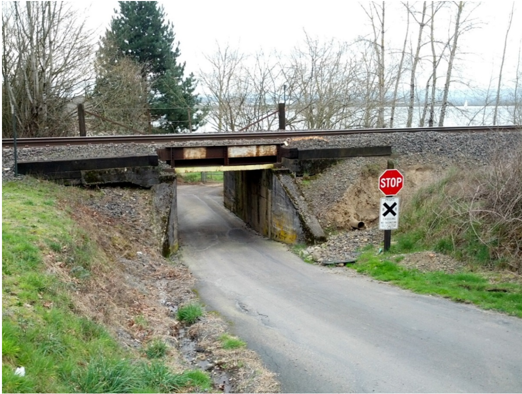
FIGURE 7-4 - UNDERGRADE CROSSING, 7' CLEARANCE
