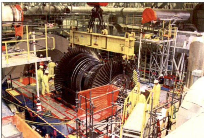
Workers install a new low pressure turbine during R-23
