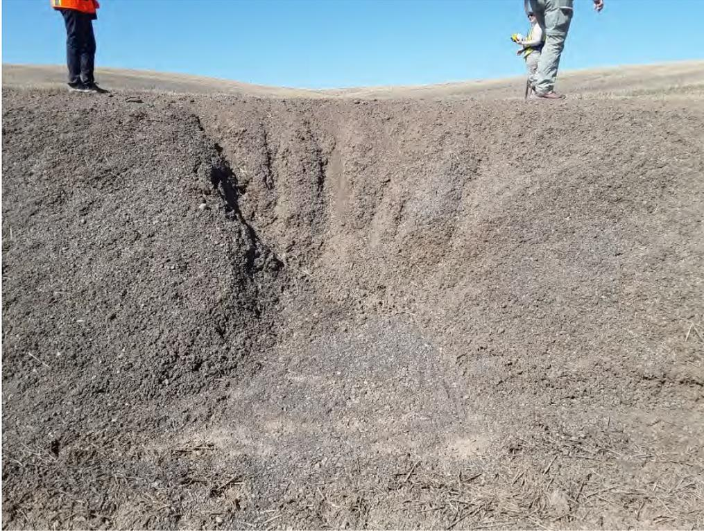
Photopoint 347. Eroded spot where culvert should be, culvert is present on opposite side of road. Facing west.
