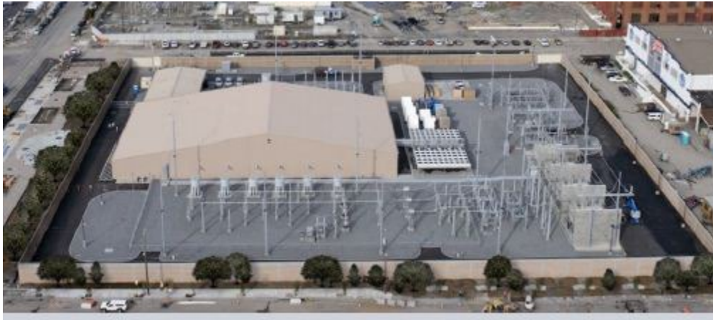
Figure 2-5. Typical Converter Station Layout
