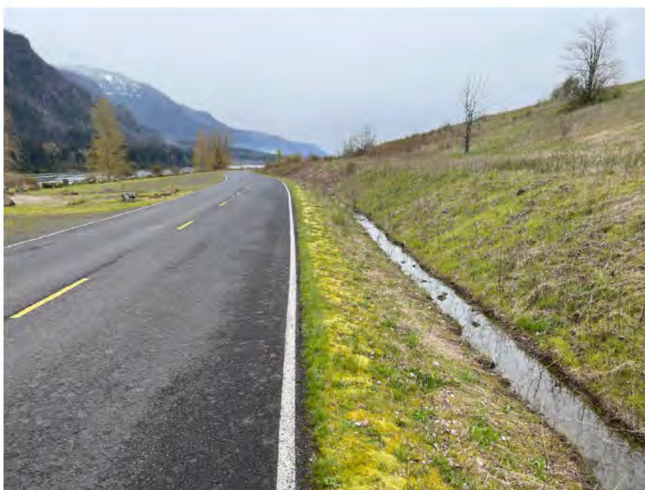
Photo 7 Overview of Ditch 2. Date: 04/20/23 Direction: Southwest
