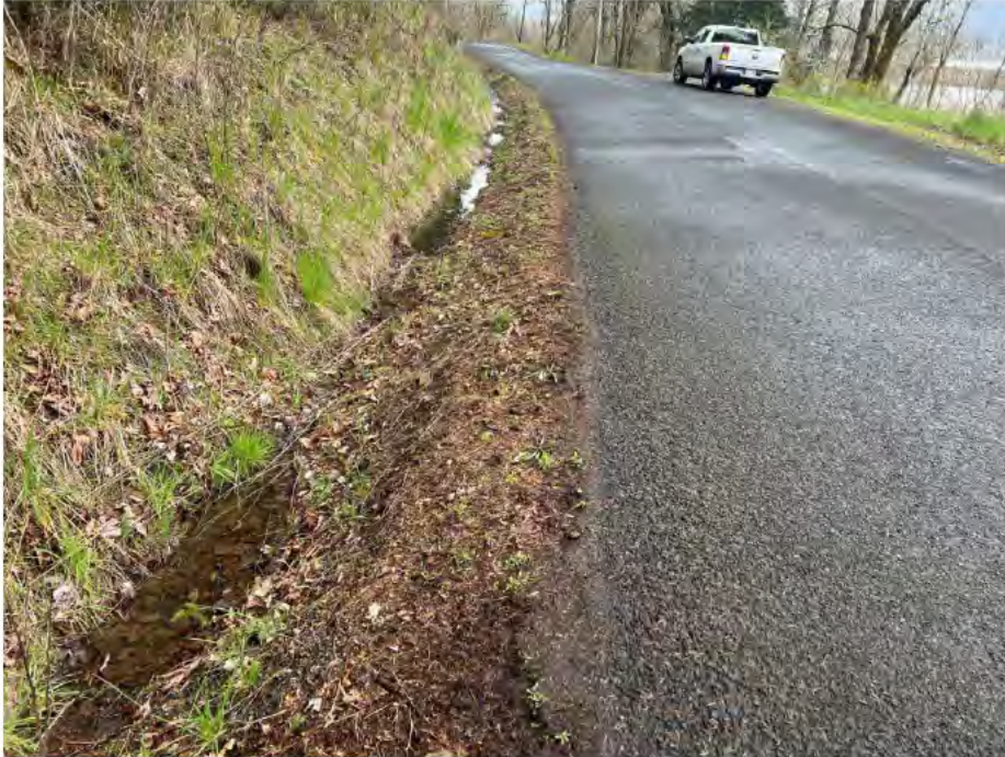
Photo 42 Overview of Ditch 6 near discharge point to culvert under Ash Lake Road. Date: 04/21/23 Direction: Northeast
