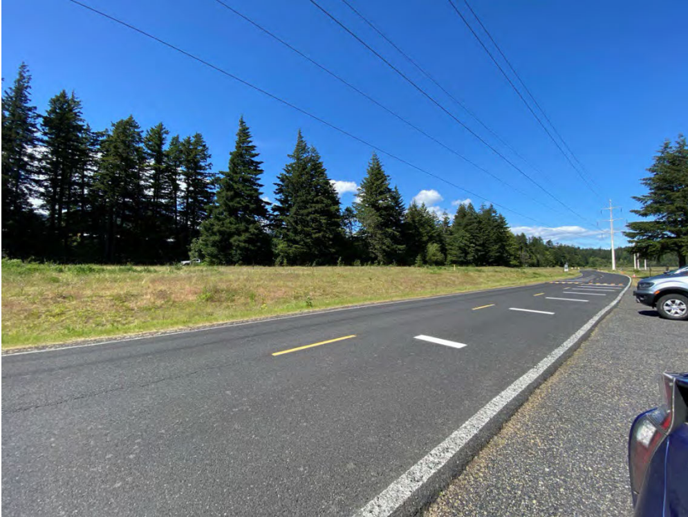
Photo 5: Looking east along Dam Access Road west of Bonneville Dam. The proposed cable route is along the north side of the road prism. May 2024.
