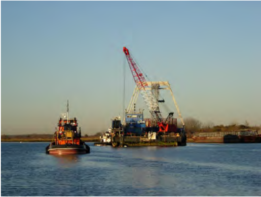
Photos of the Neptune Project (clockwise from top left): The installation barge laying cable in New Jersey's Raritan River; conduit for installation of the DC land based cable is laid in trenches along the Wantagh Parkway on Long Island; the street view of Neptune's converter station in Sayreville, New Jersey and the interior view of the converter valve hall.
