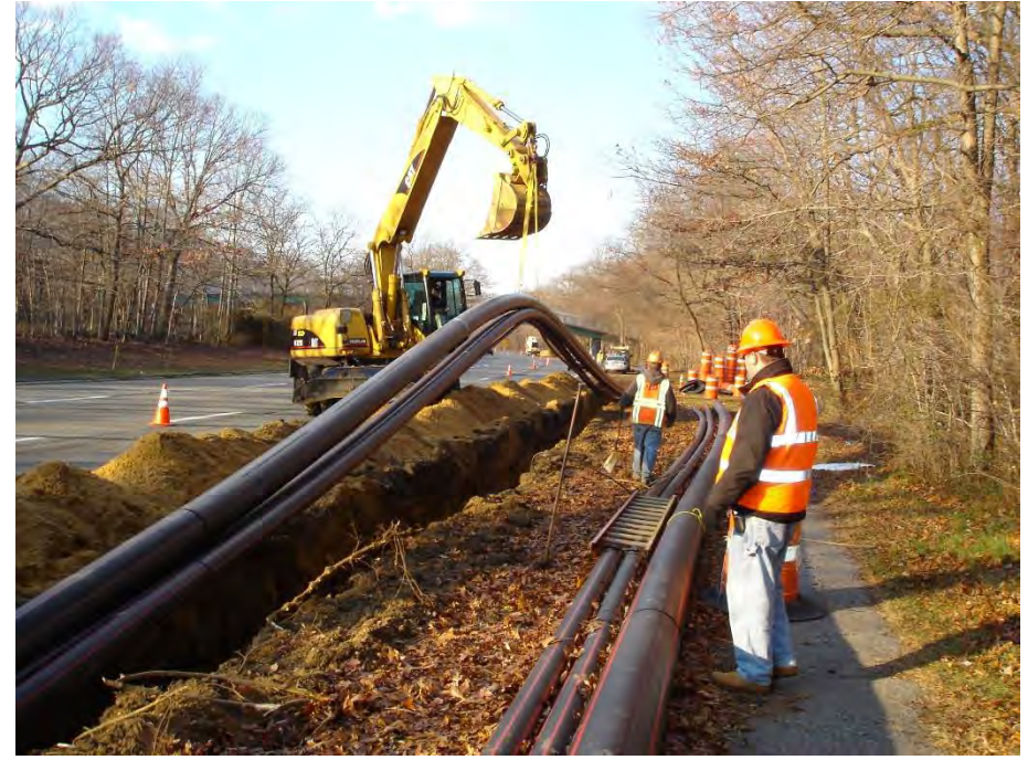
Photos of the Neptune Project (clockwise from top left): The installation barge laying cable in New Jersey's Raritan River; conduit for installation of the DC land based cable is laid in trenches along the Wantagh Parkway on Long Island; the street view of Neptune's converter station in Sayreville, New Jersey and the interior view of the converter valve hall.
