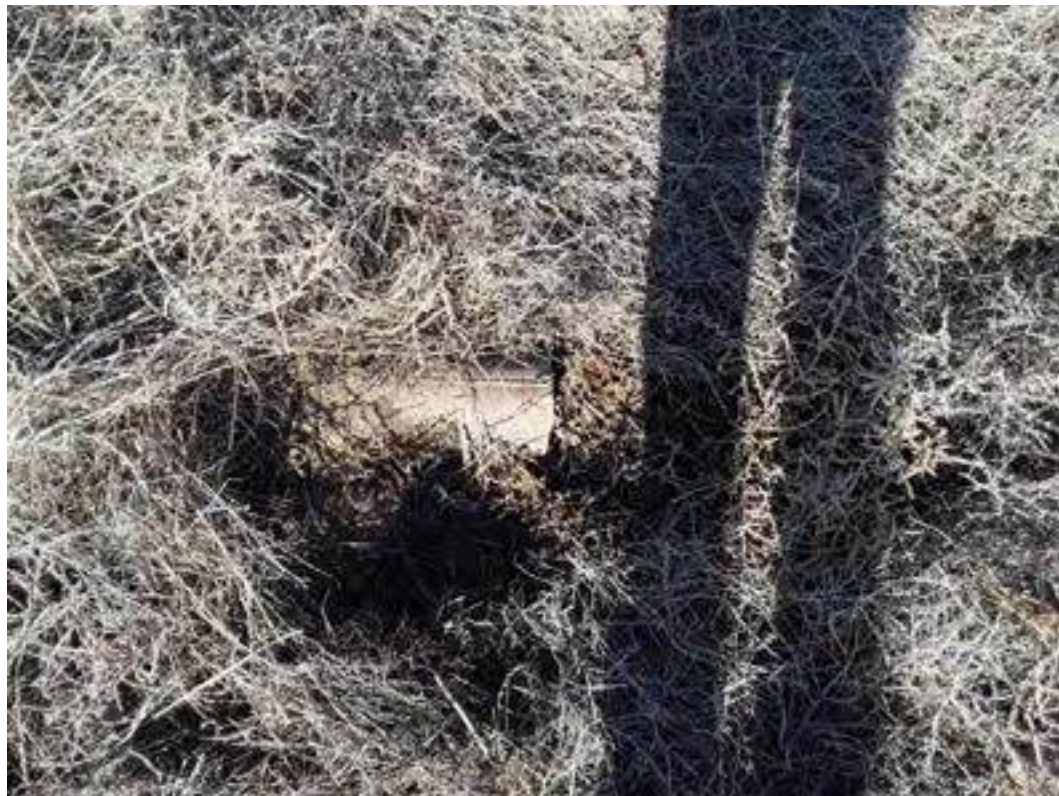
Photopoint 4011. Pipe into livestock pond. PD401. Facing west.
