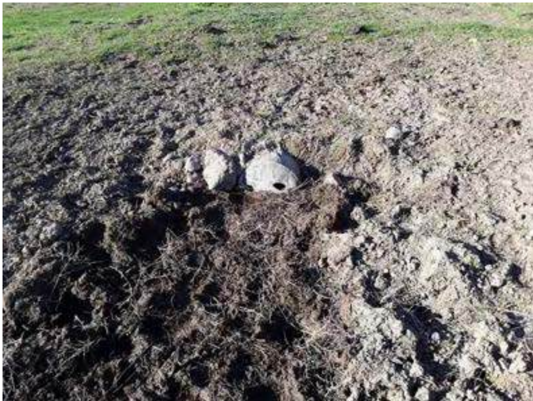
Photopoint 4001. Pipe into livestock pond. PD400. Facing southwest.
