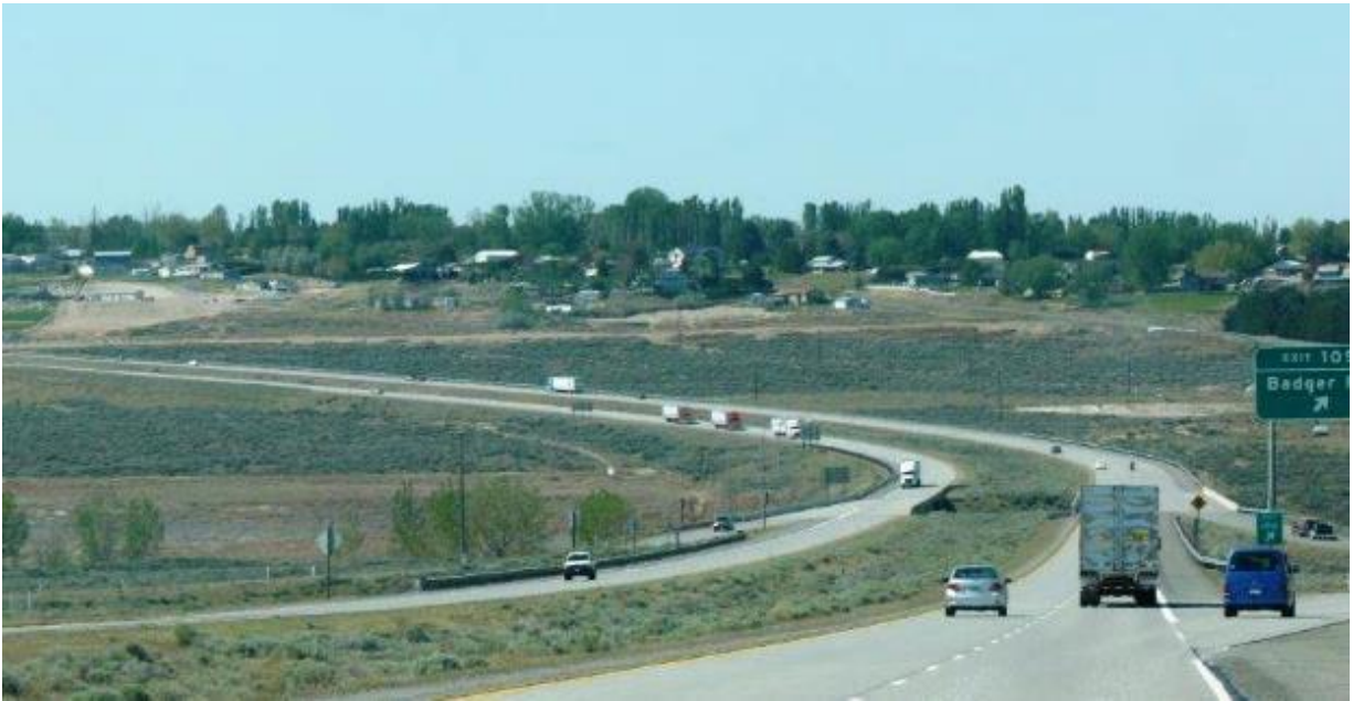
Highway transportation facilities along Interstate 82 and Badger Road
