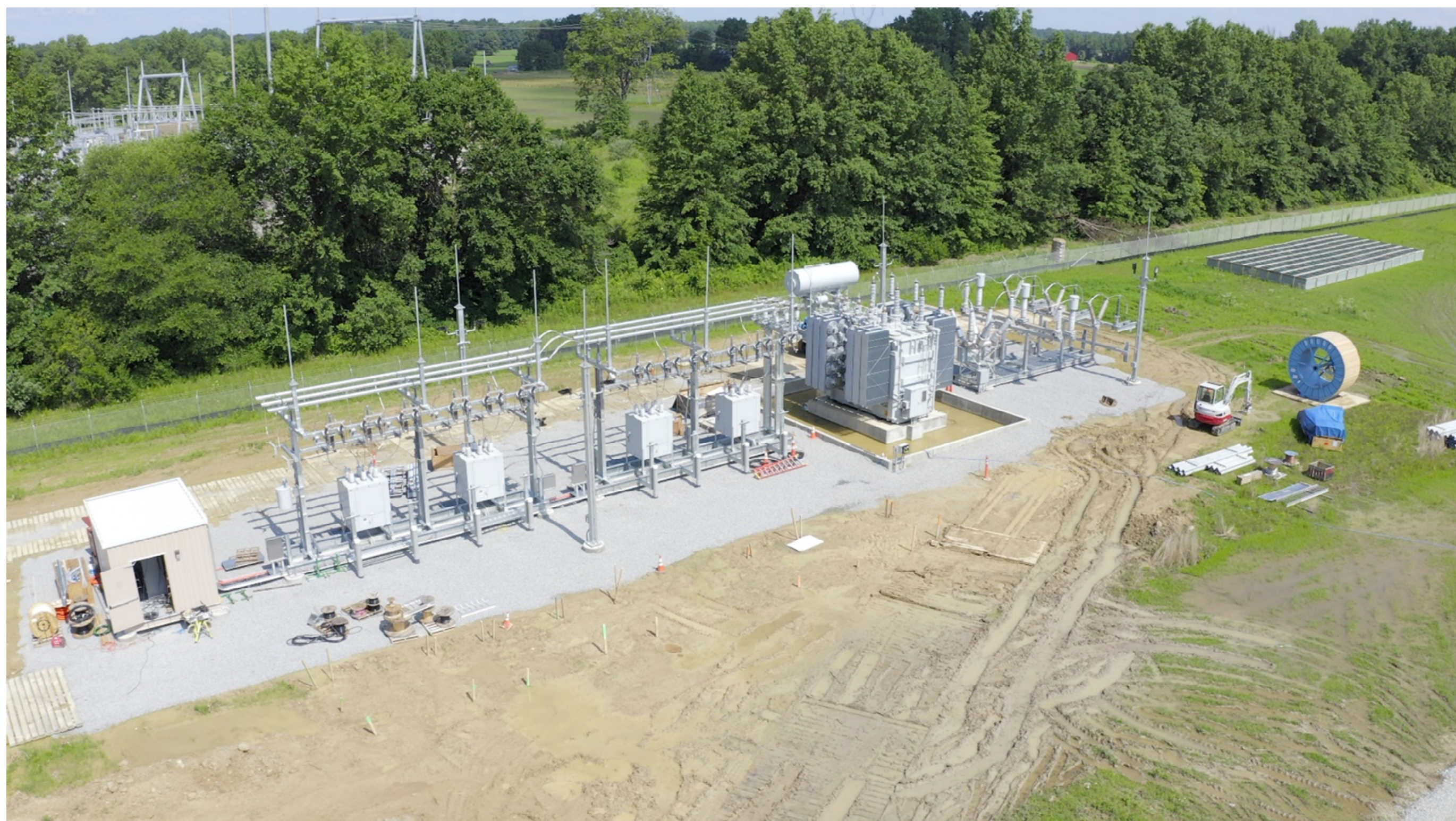
Construction of the substation
