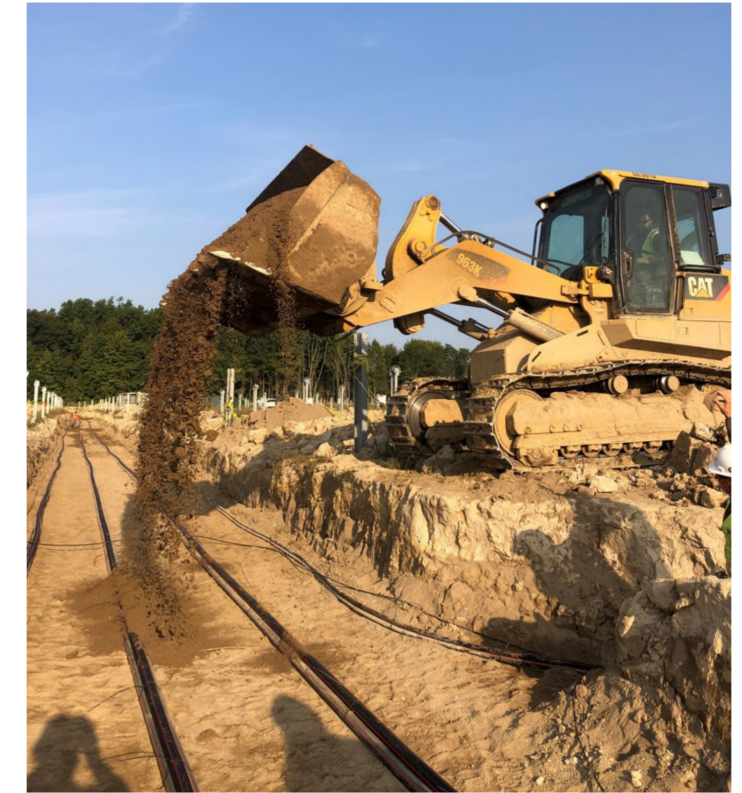
Trenching and installation of buried electrical cables
